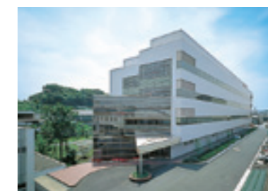
POLA Yokohama Research Center
