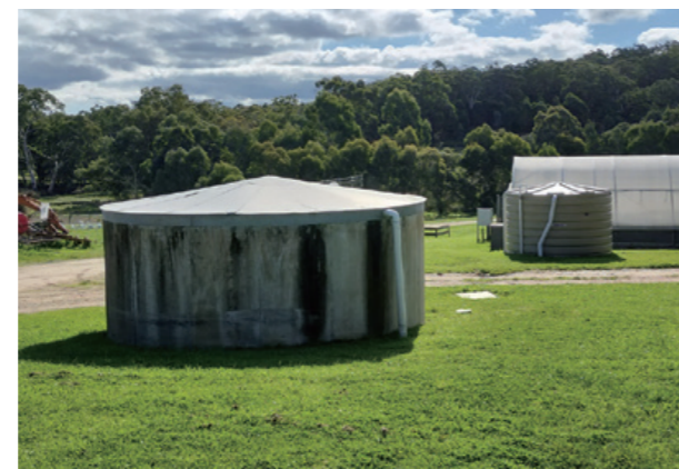
Jurlique: Flame-retardant tanks to store rainwater
