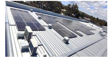
The solar power generation system at Jurlique's Adelaide factory
