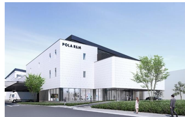
Technical Development Center
